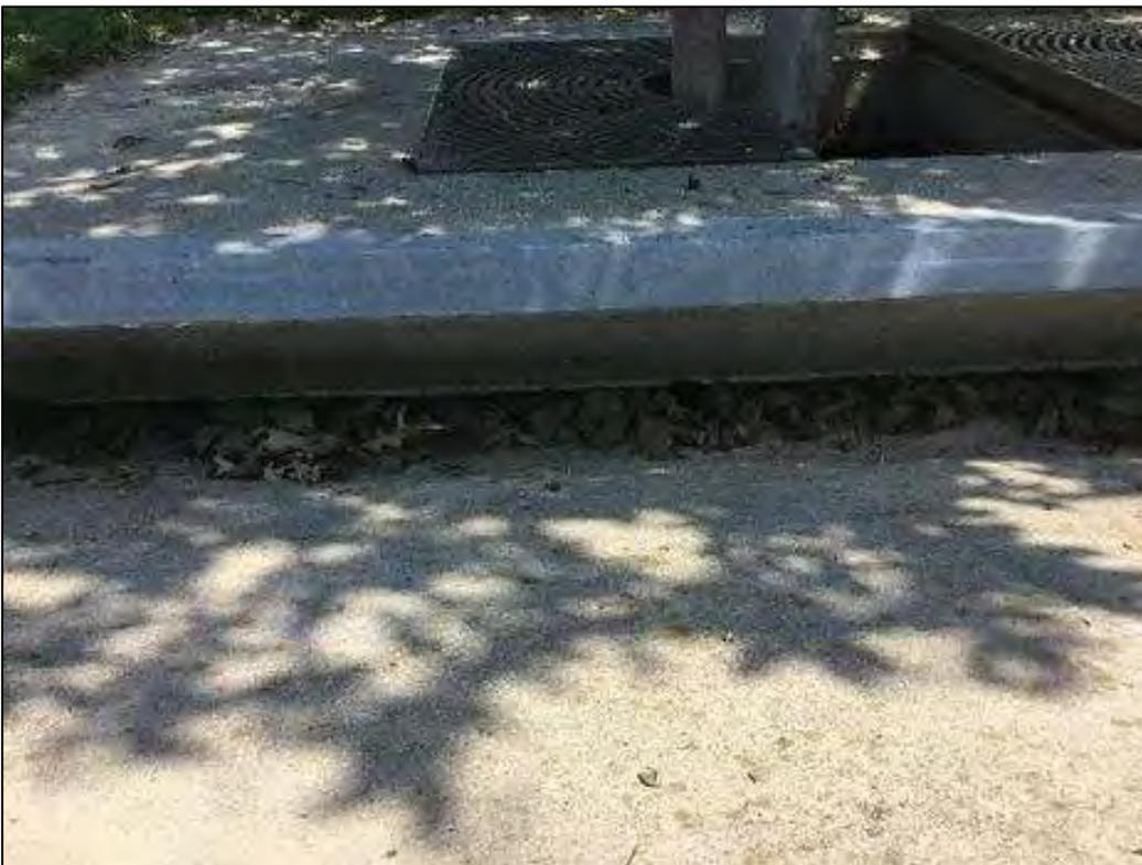
Close-up of partially blocked curb inlet throat
