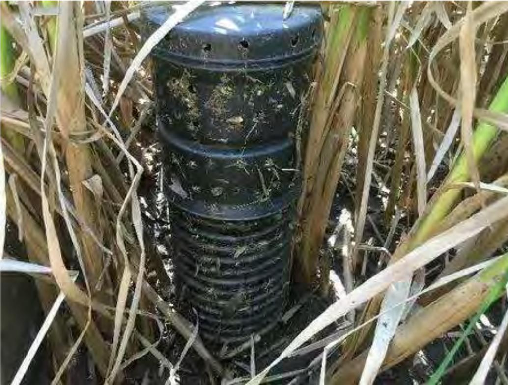
Riser with low-flow orifices
