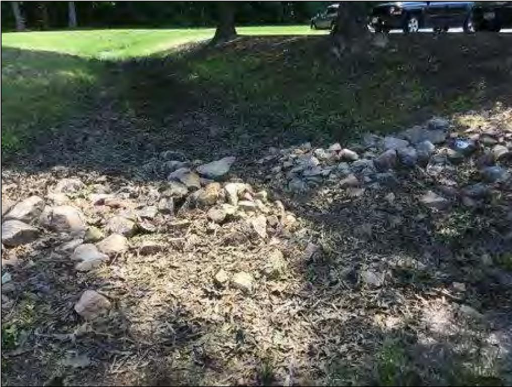
Sediment accumulation on riprap
